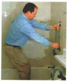
**Test-driving the installation.** When he has completed an installation, the author always checks his work by putting his weight on the bar and giving it a few good pulls.
